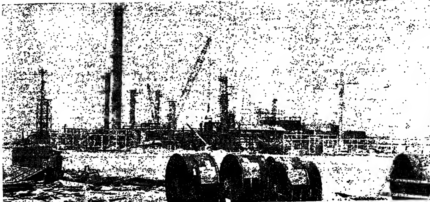
Qatar's first petrochemical plant under construction at Umm Said. It is scheduled for completion by 1980
